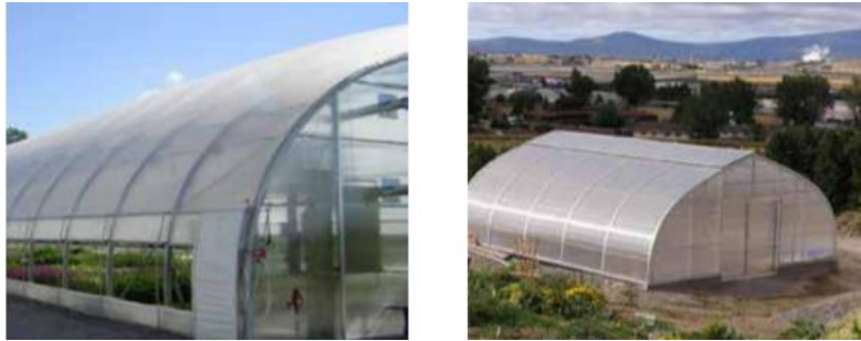
Figure 2.11 Recouvrement de serres
